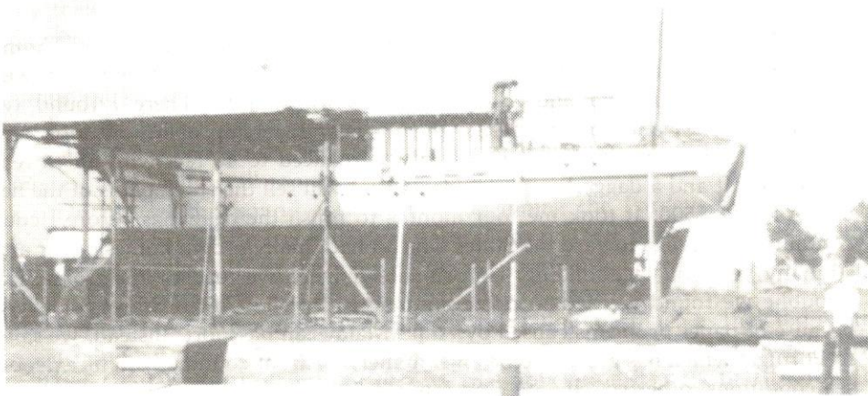
Sri Dewi showing her east side, installing deck super structure.
